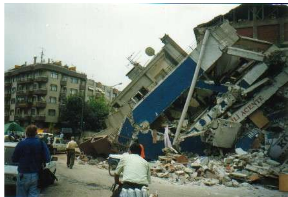
Picture 4: Demolished Building
