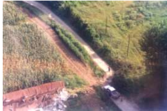
Picture 2: Lateral Shift in Road
