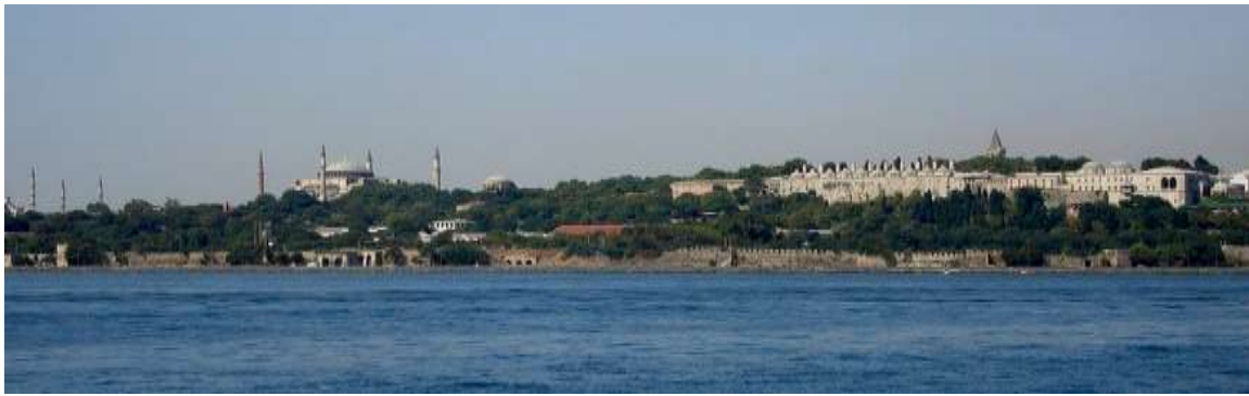
Picture 3: Topkapı Palace
